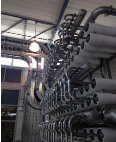
Figure 26 – A set of membranes through which brackish water passes known as a treatment train (Photo Credit: William Delgado-Thompson)
