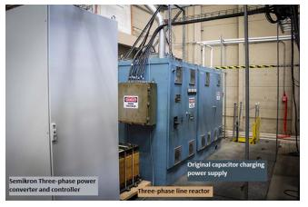
Fig. 11. Full-scale CCPS with inverter and three-phase line reactor.
