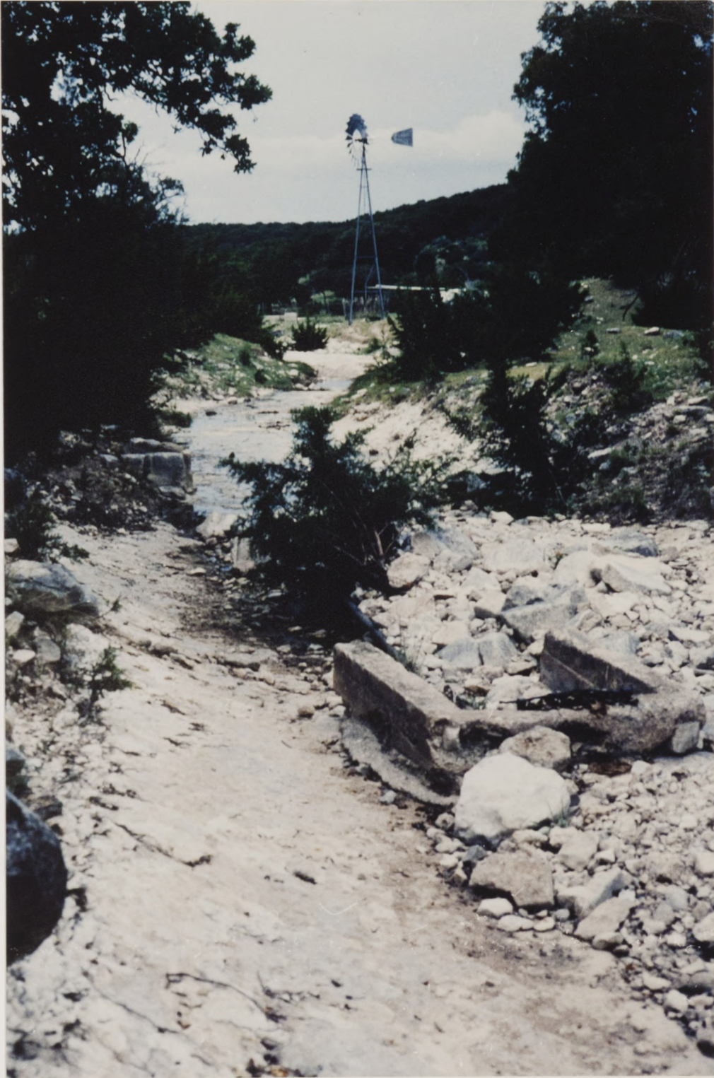
Figure 24. The concrete structure in the foreground was designed to capture and pipe spring water to a cattle reservoir. Reduced spring flow to this structure in recent decades, possibly due to the growth of phreatophytes, and the associated increased evapotranspiration, necessitated the drilling of a well.
