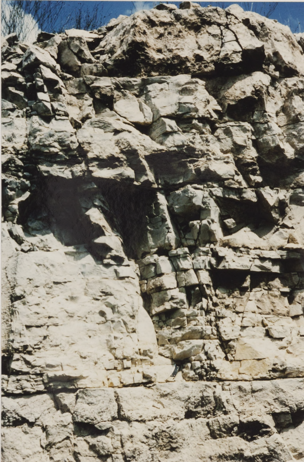
Figure 22. Hydraulically connected fractures and horizontal bedding planes in the Edwards Group serve as conduits for flow in the unsaturated and saturated zones. A pocket knife at the bottom center of the photograph serves as scale.
