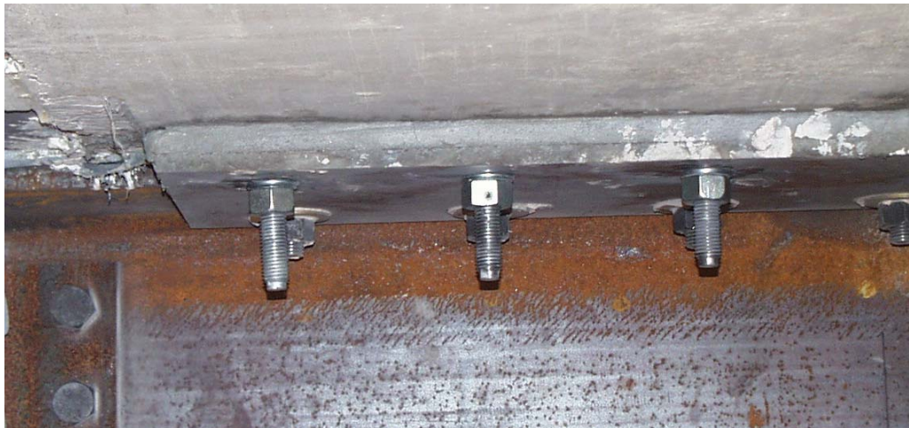
Figure 6.68 Threaded rods bolted to plate
