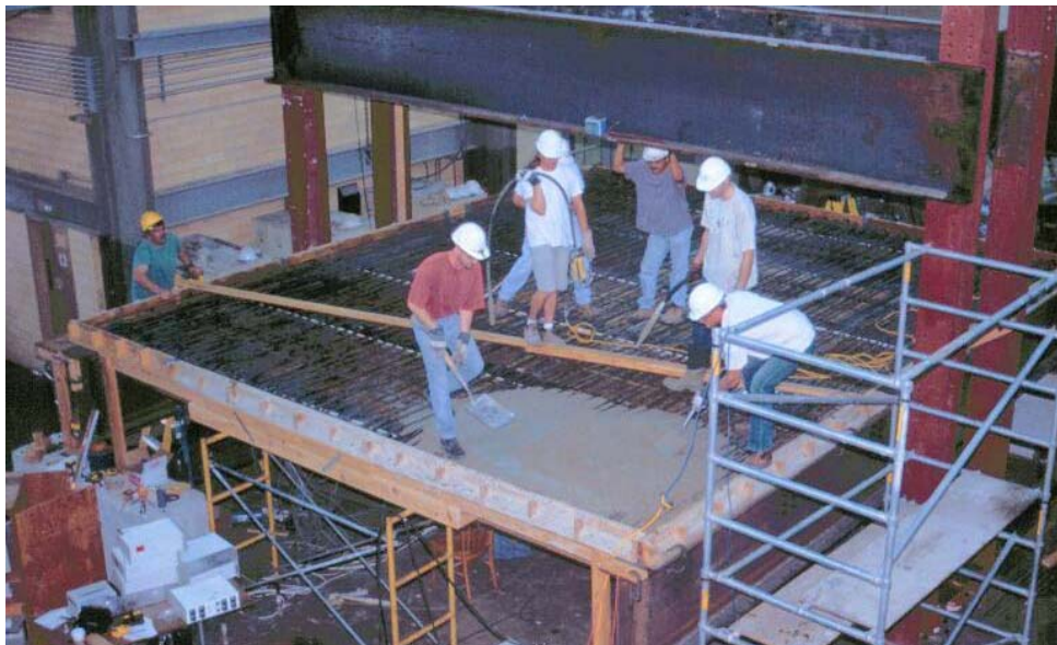
Figure 6.12 Concrete pour and finishing
