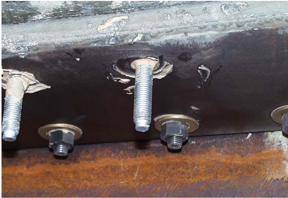
Figure 6.67 Threaded rod installed in slab with epoxy
