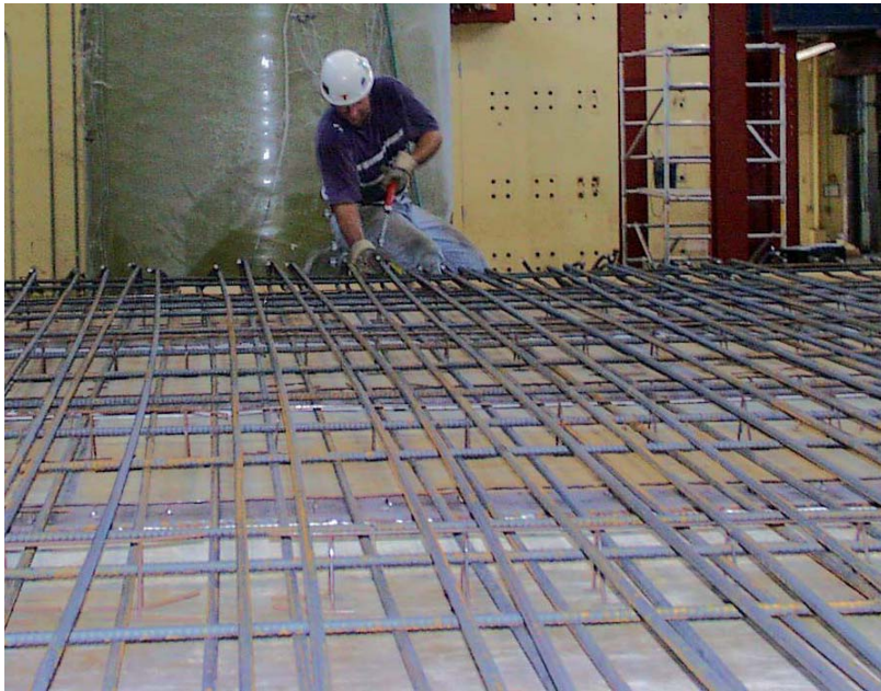
Figure 6.11 Reinforcing bar placement in slab
