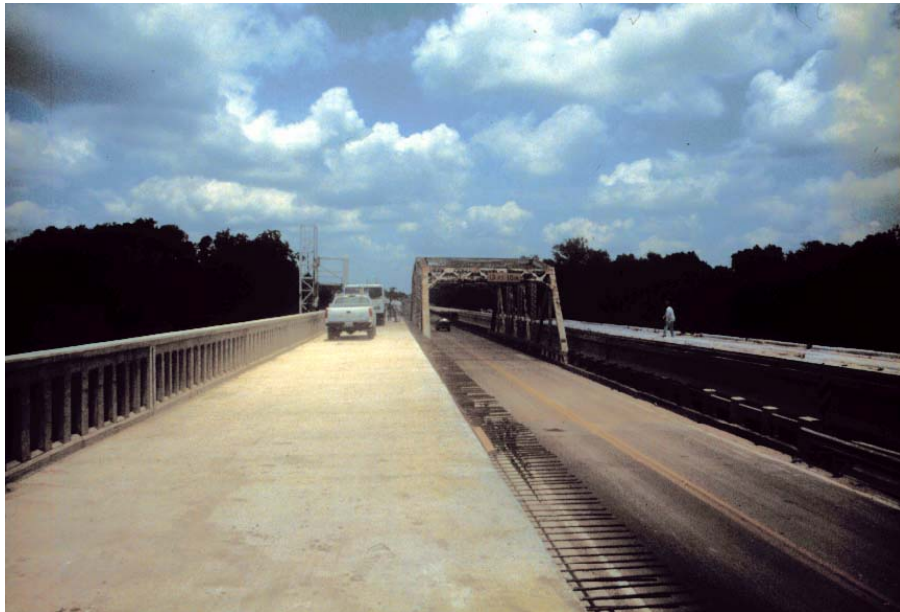
Figure 5.2 Lanes built around the original bridge
