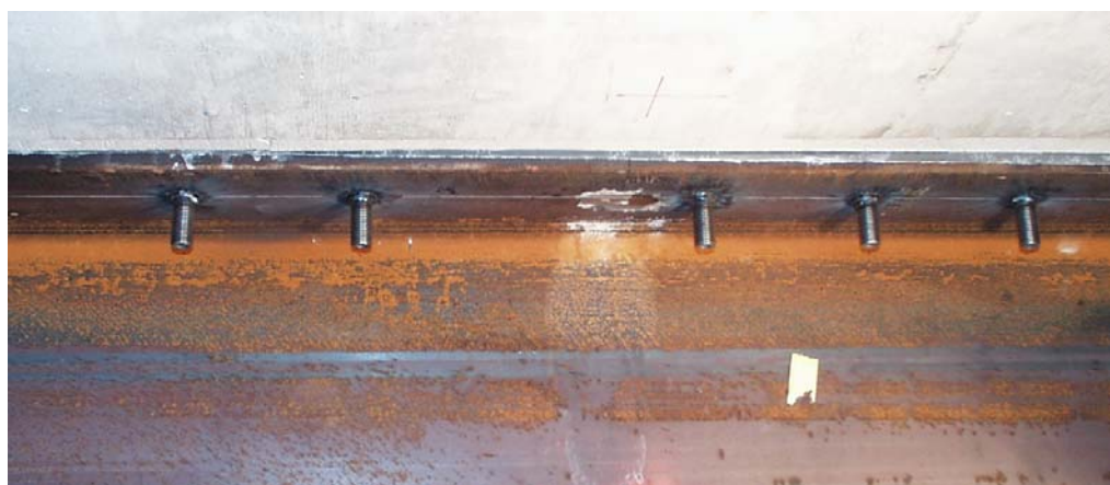
Figure 6.63 Threaded studs welded to the inside top flange of the transverse beam
