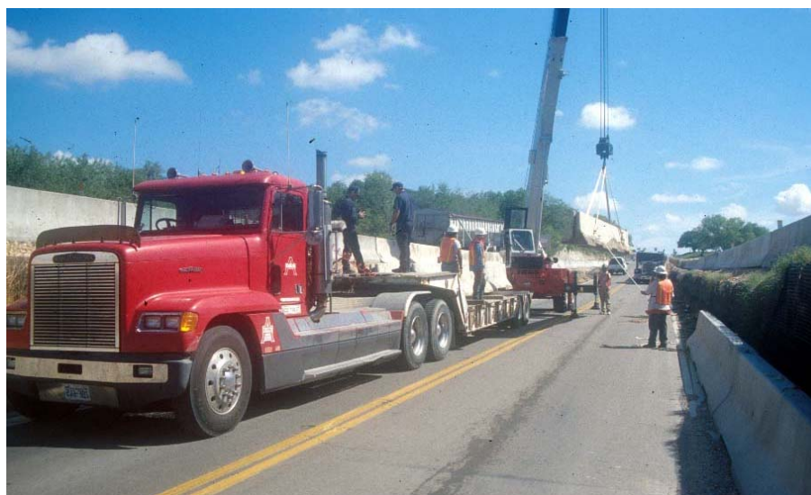
Figure 5.20 Barrier loading to increase axle weight
