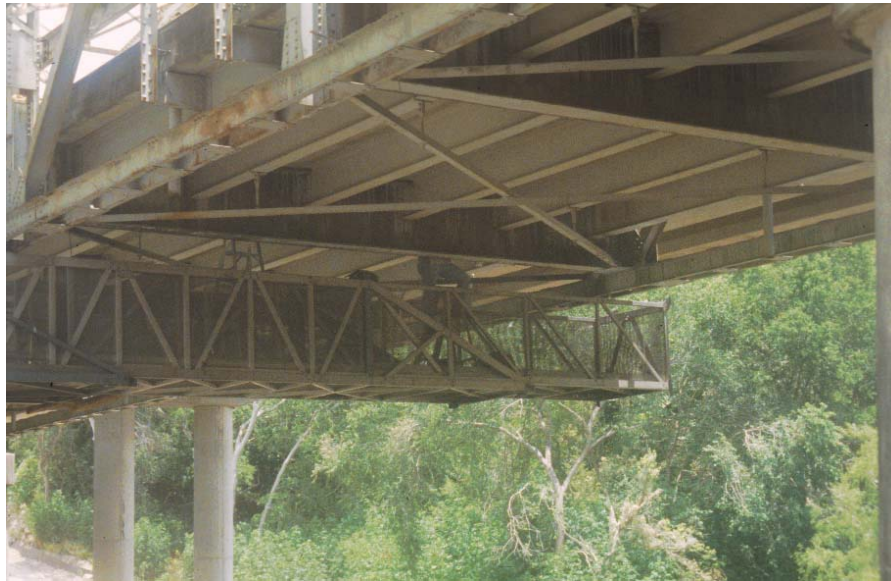
Figure 5.14 Platform extension used to instrument deck
