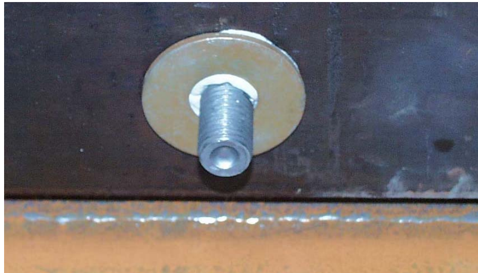
Figure 6.77 Washer covering epoxy filling
