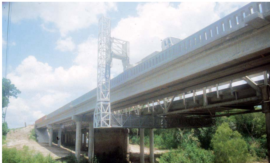
Figure 5.13 Access to bridge deck
