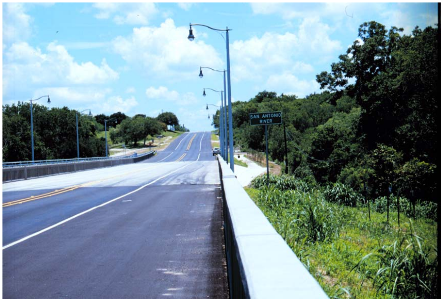
Figure 5.5 South view of finished replacement bridge
