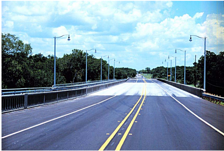
Figure 5.4 View to the north of finished replacement bridge
