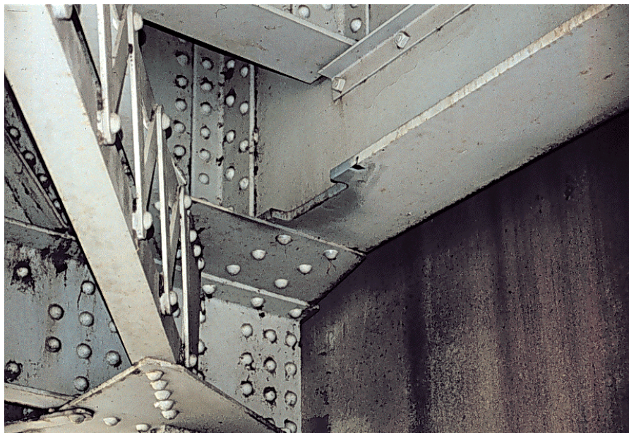
Figure 2.16 Location after steel sample removal
