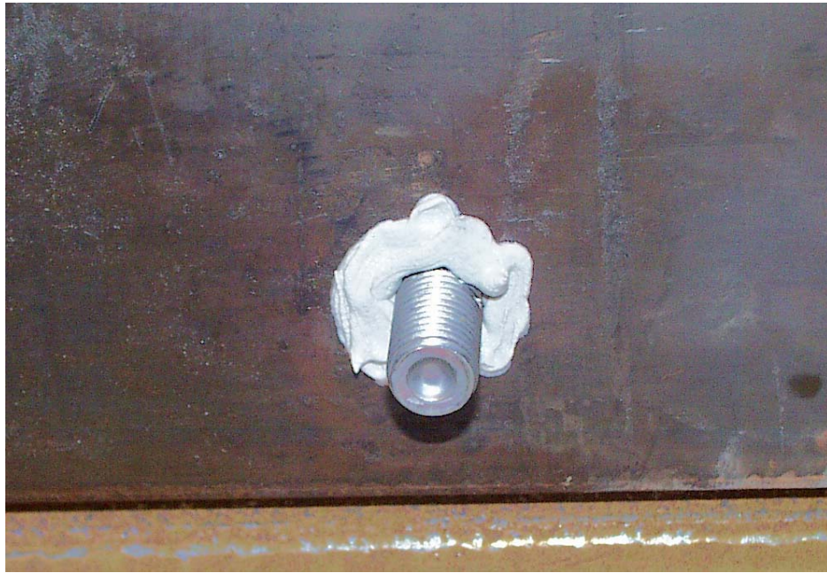
Figure 6.76 Gap filled with HSE 2421 epoxy
