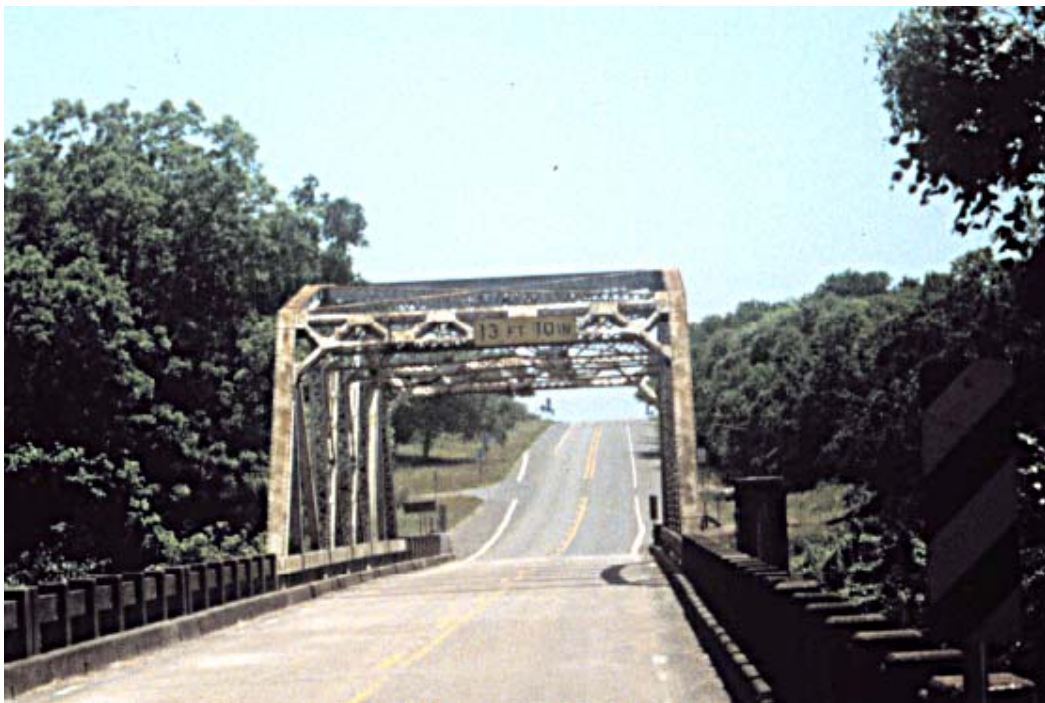
Figure 5.1 Parker truss bridge in Goliad, Texas
