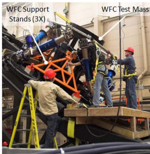
Figure 11. WFC test mass installation
