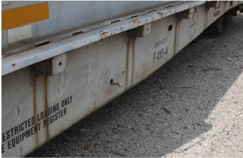
Figure 11.7: Lower position valve, line-of-sight is completely obstructed
