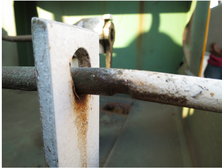
Figure 2.1: Bleed Rod with worn notch
