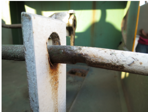
(a) Rod notch in San Antonio Yard
