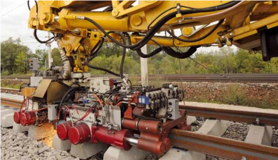
Figure 2-7: Plasser & Theurer APT 1500 R rail welding robot [P&T, 2013]
