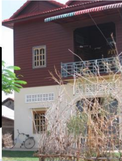
Photo 4: An "ideal" home in Chanleas Dai; concrete on bottom with a wooden second story and tiled roof.
