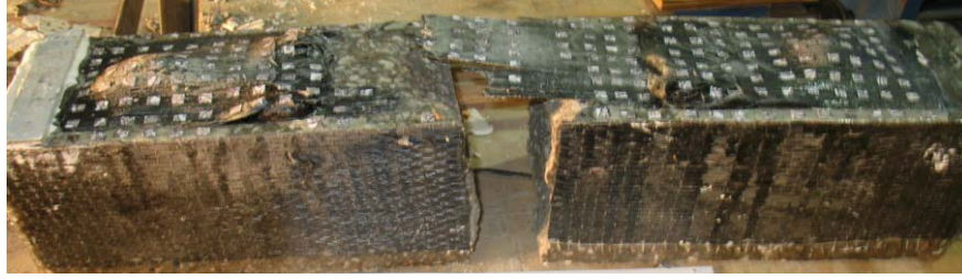
a) Rupture of CFRP strengthening sheet
