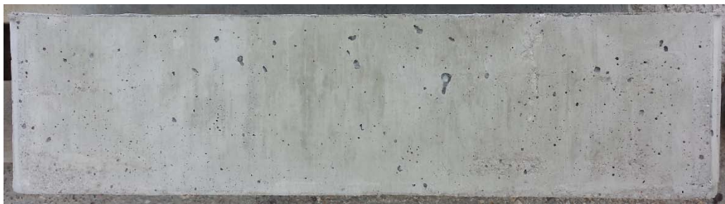
Figure 3.7 Concrete surface before grinding
