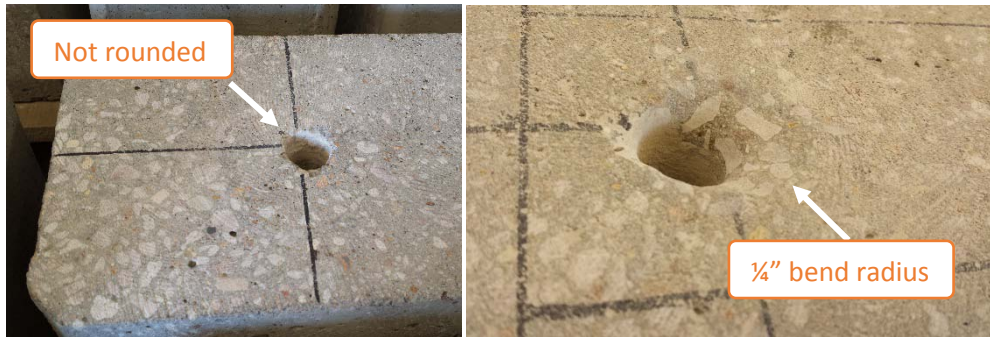
Figure 3.10 Rounded anchor hole
