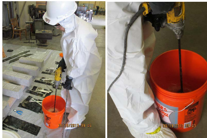
Figure 3.18 Mixing Tyfo® S Epoxy
