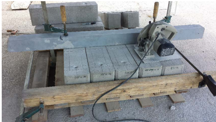
Figure 3.11 Preparing to saw a 1 in. notch in beams
