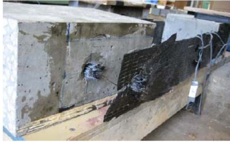
b) Rupture of CFRP anchor
