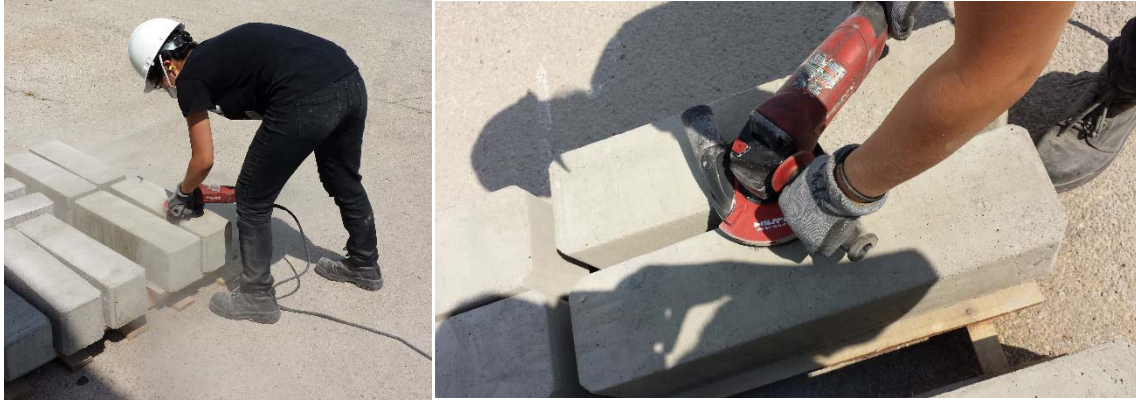
Figure 3.6 Grinding concrete surfaces to prepare for CFRP installation
