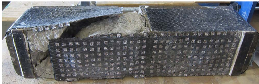
d) Concrete fracture behind anchor
