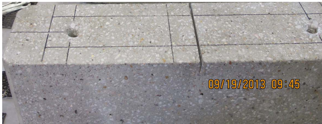
Figure 3.8 Concrete surface after grinding
