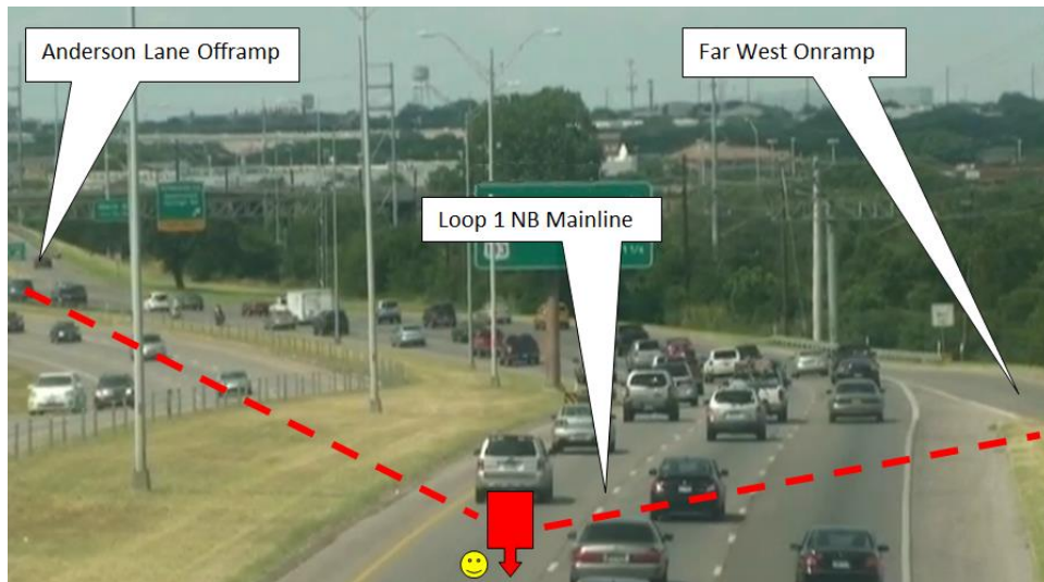
Figure 5.6 - View From Bridge
